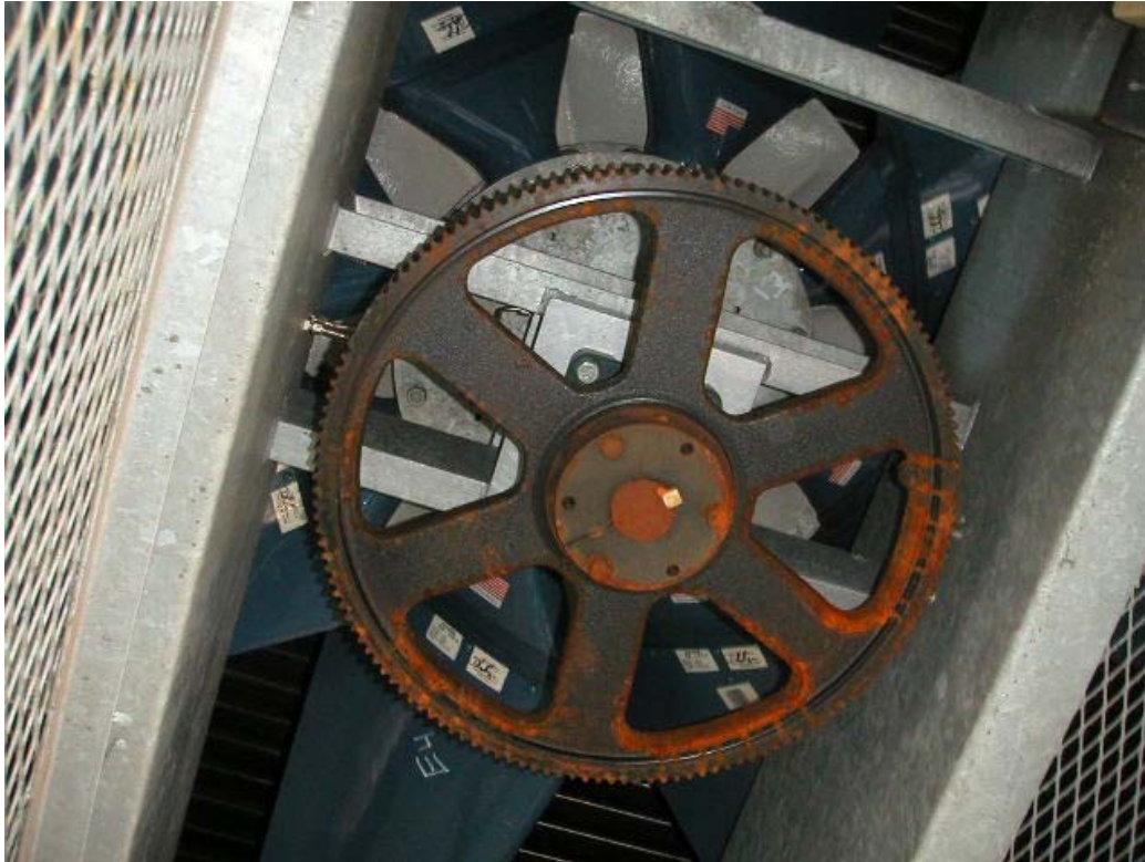
Figure 3.2. Fan and driven sprocket viewed from below
