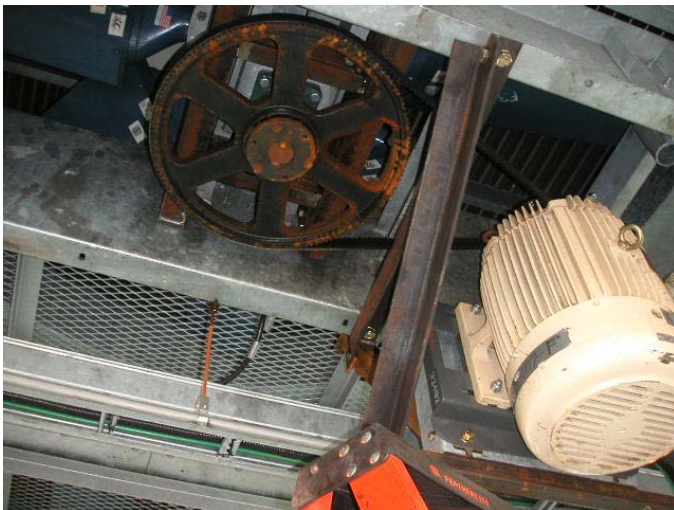
Figure 3.4. Braces in the north-south direction.
