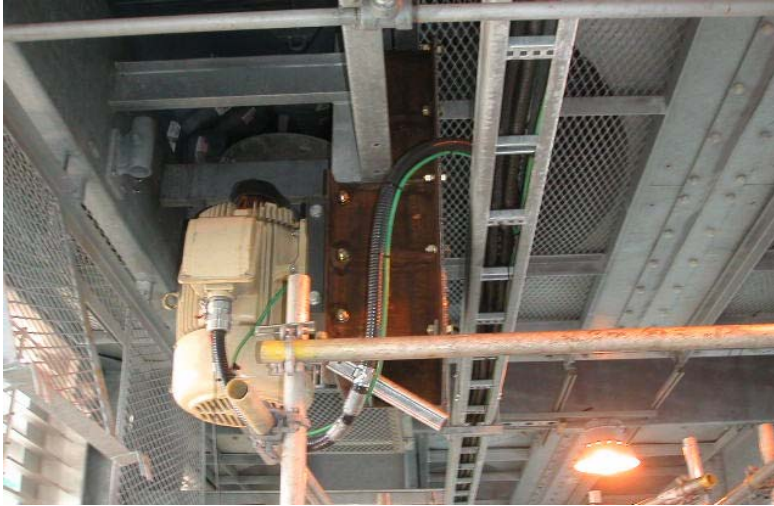
Figure 3.5. Looking west at the rotationally stiff brace on motor D
