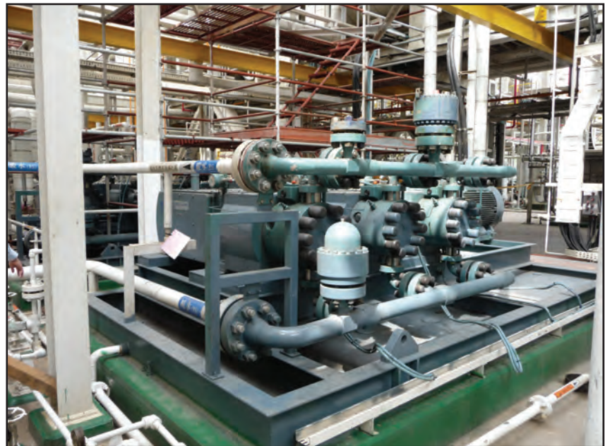
Photo 1. Reciprocating diaphragm pump
