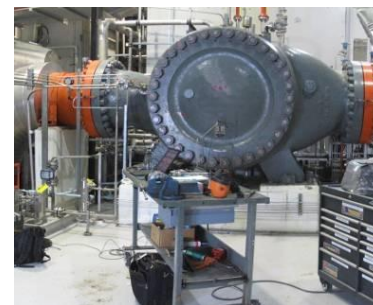
Troubleshooting support at gas pipeline facility
