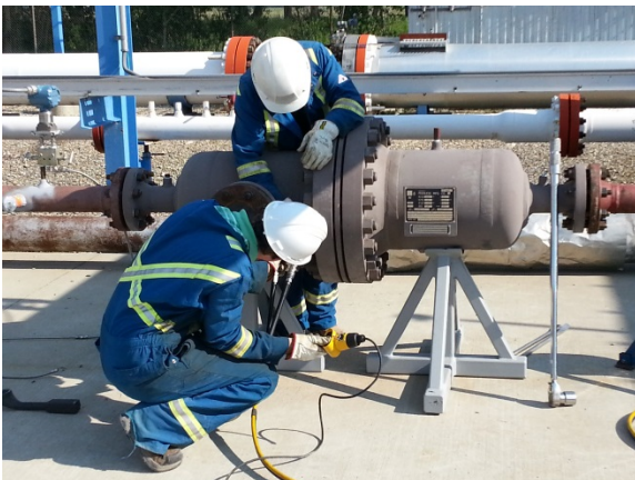
Customized Pulsation Bottle (donated by Peerless Manufacturing)
