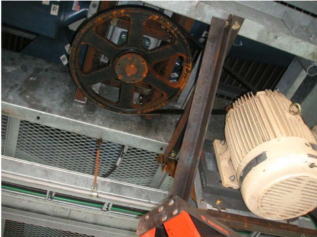
Photograph 3: The photograph above shows one side of the bracing. The stiffening was primarily in the north-south direction.
