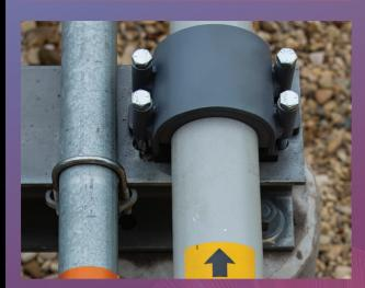
DamperX<sup>TM</sup> damper clamp: field testing has proven a 40 - 90% vibration reduction compared to conventional clamps.
