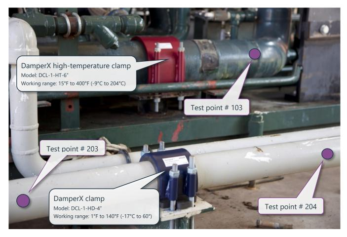
Figure 5 – Main discharge pipe with DamperX clamps installed (TPs #203 and #204)
