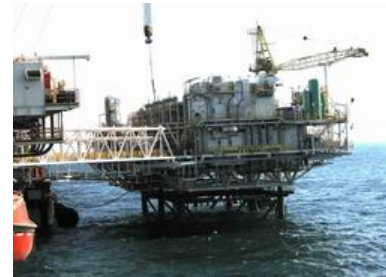
Structural dynamic analysis for Bunduq Platform (Abu Dhabi) including 5 large compressor packages (20,000 HP)
