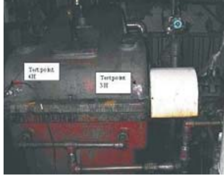
Picture 1: High speed side of the box, Test Points 3 and 4: (Turbine to the right)
