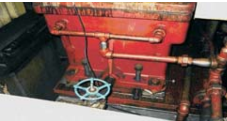
Picture 4: Gearbox base on the south side.
