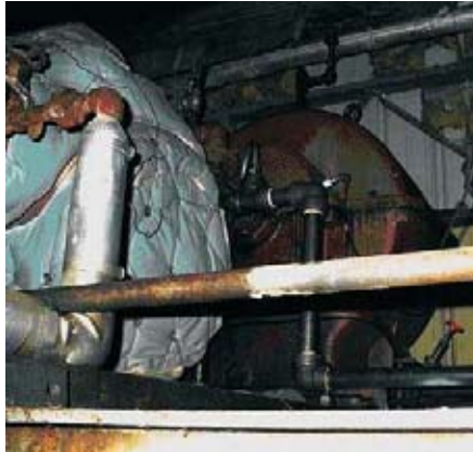
Picture 2: View of Test Point 5 with accelerometer mounted with stud on nut glued to box in Horizontal orientation. The oil pump is on the turbine side of the low speed shaft.
