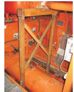
Figure 6: Inlet flange Vertical support with cross braces
