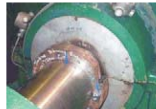
Figure 8. Shaft balance ring installed between the turbine and generator.
