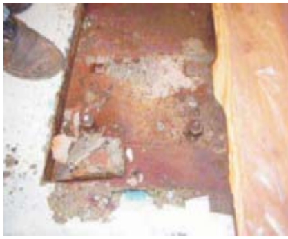
Fig. 9 & 10. Two views of grout under the generator DE bearing pedestal as found in the spring 2003.
