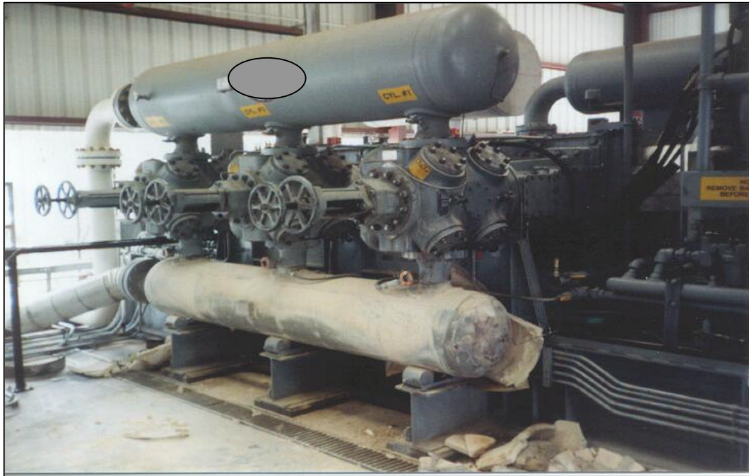
Figure 1: Residue Gas System
