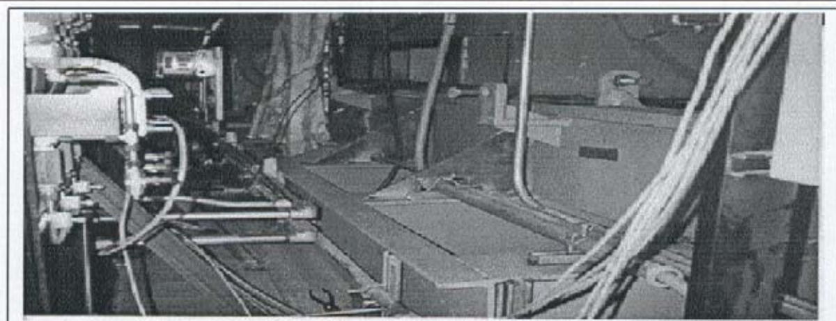
Picture 6: External Gussets added to motor pony skid
