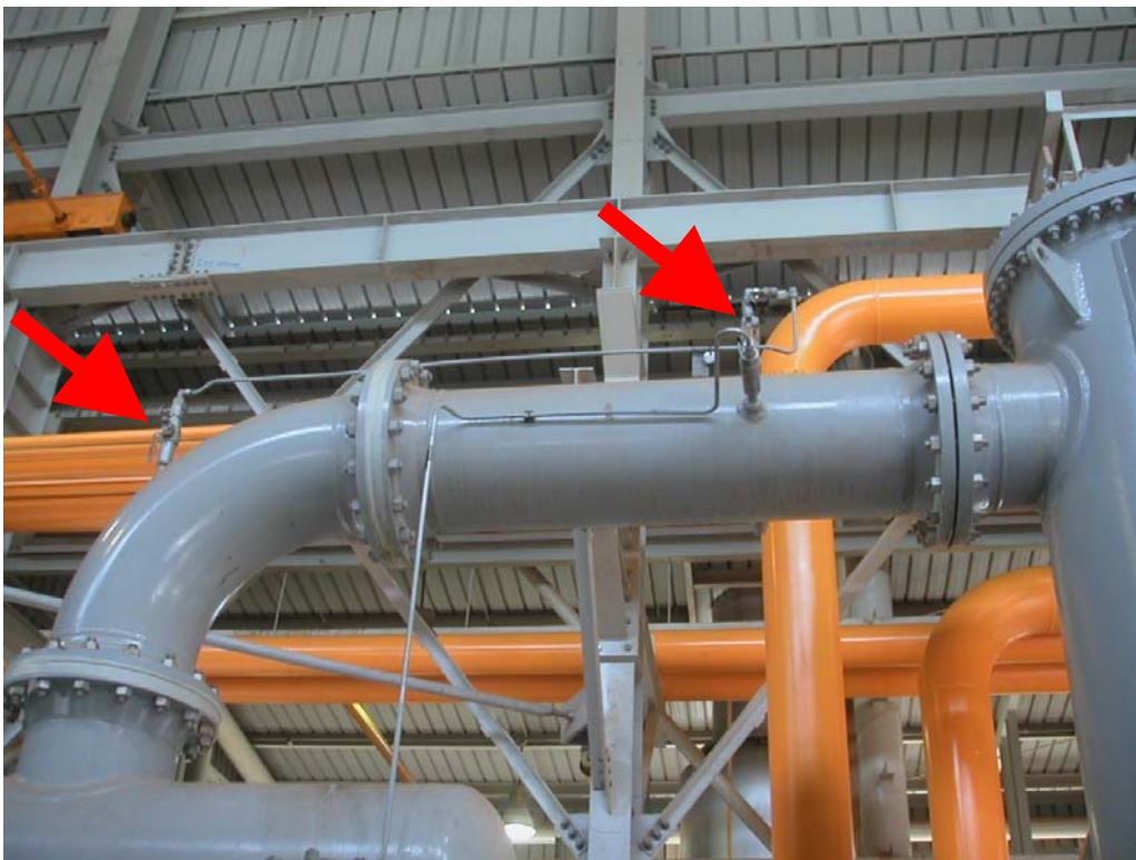
Picture 2 More small bore attachments.
