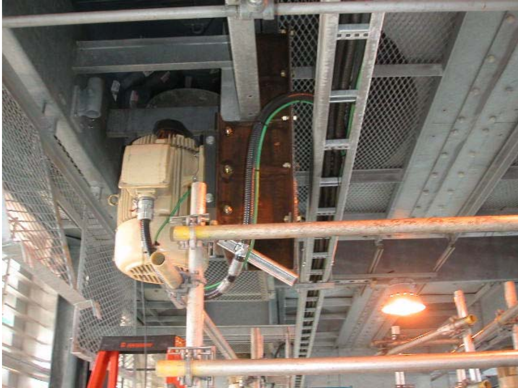
Photograph 4: Looking west at the rotationally stiff brace on motor D
