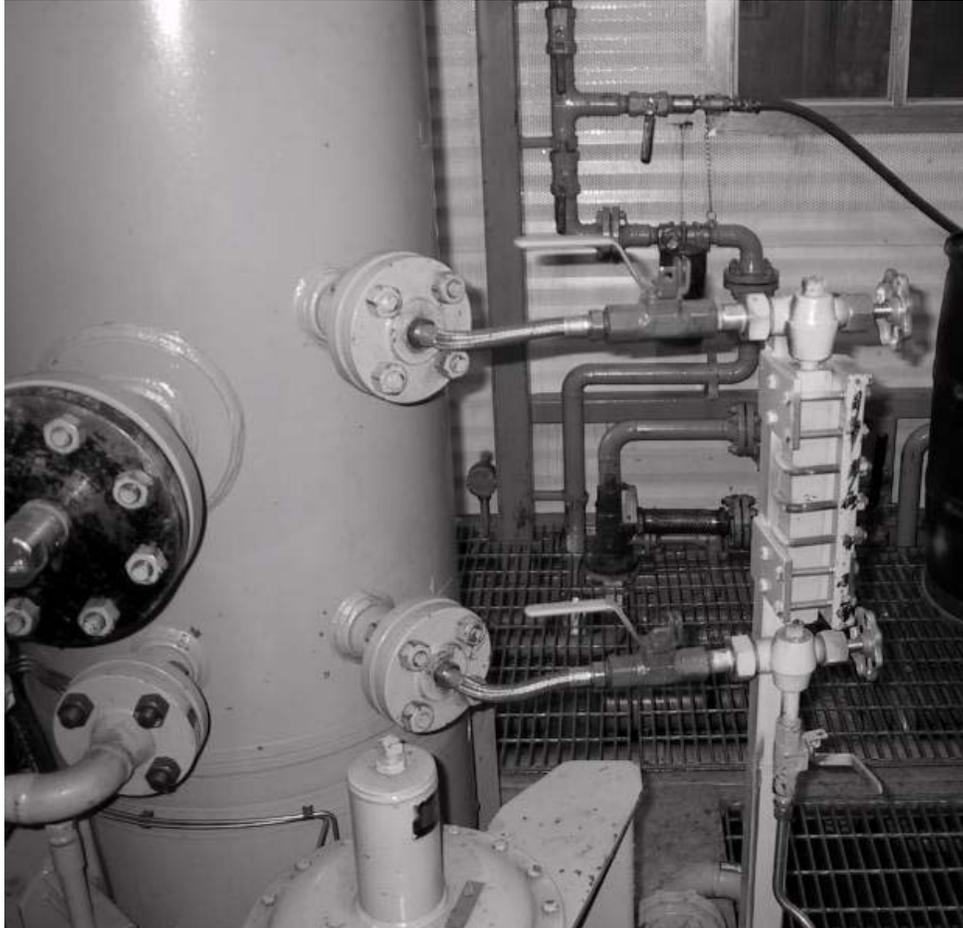
**Figure 4. Example of Remote Mounted Sight Glass Connected to Scrubber with Tubing**
