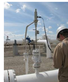
Vibration Audit on Small Bore Piping
