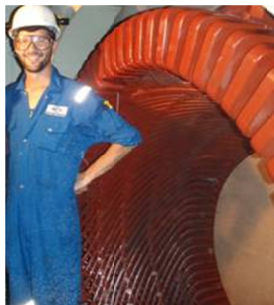
Turbine end of generator stator
